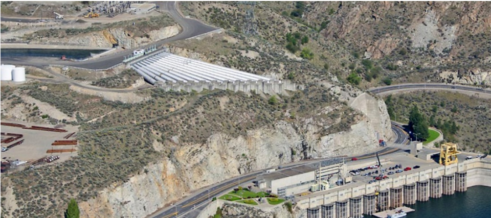
Pic 1: Grand Coulee Dam Pump Generating Plant
