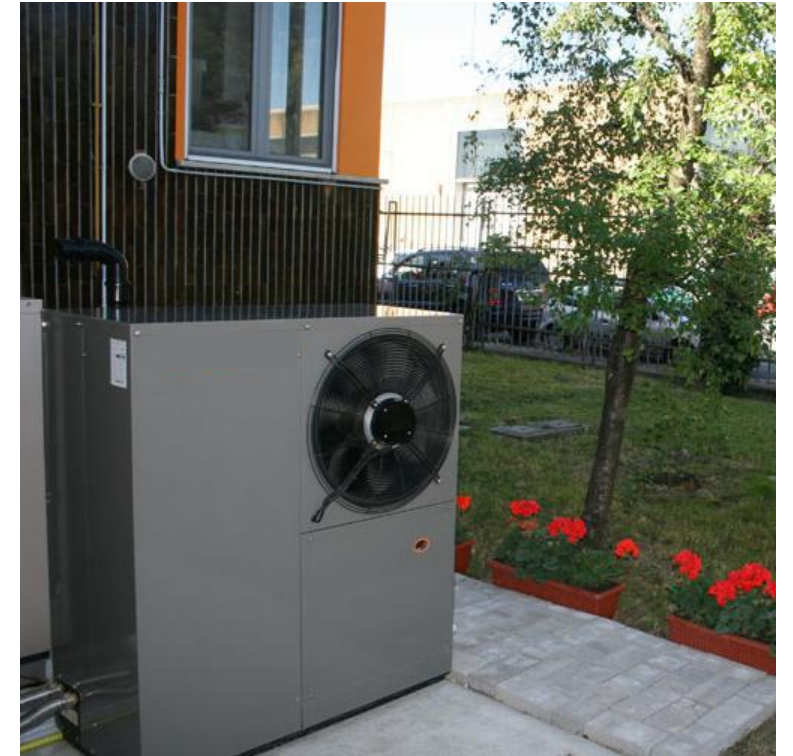
GAHPs commercially available in EU for home heating, in 2016 an 18 kW (61 MBH) output released by Italian mfr. Unit costs are prohibitive for US, > $11,000 (excl. shipment)
