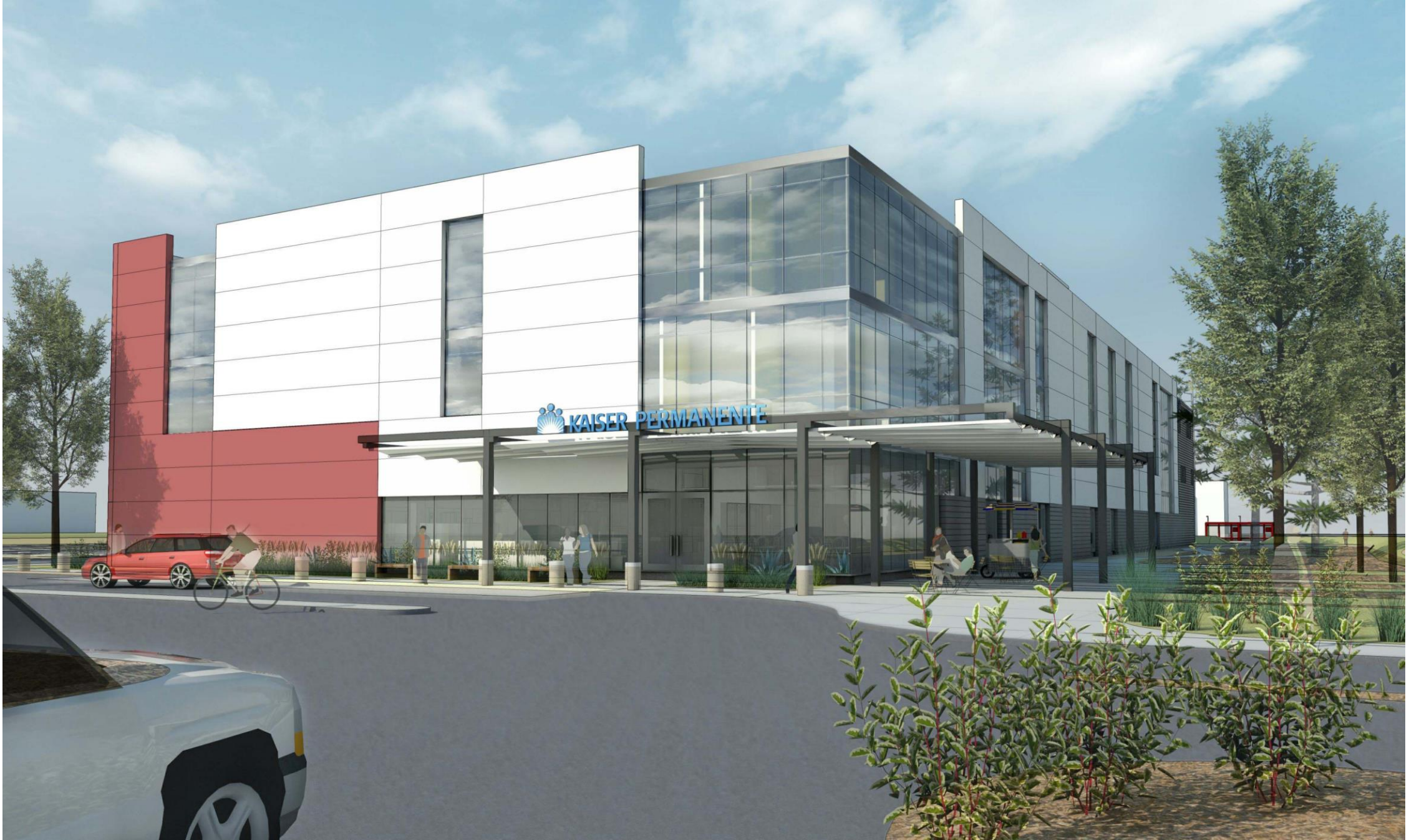
KAISER PERMANENTE MEDICAL OFFICE BUILDING
